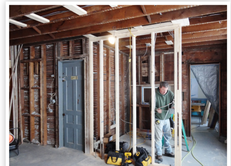
Electric lines being installed in Main Lodge kitchen.
